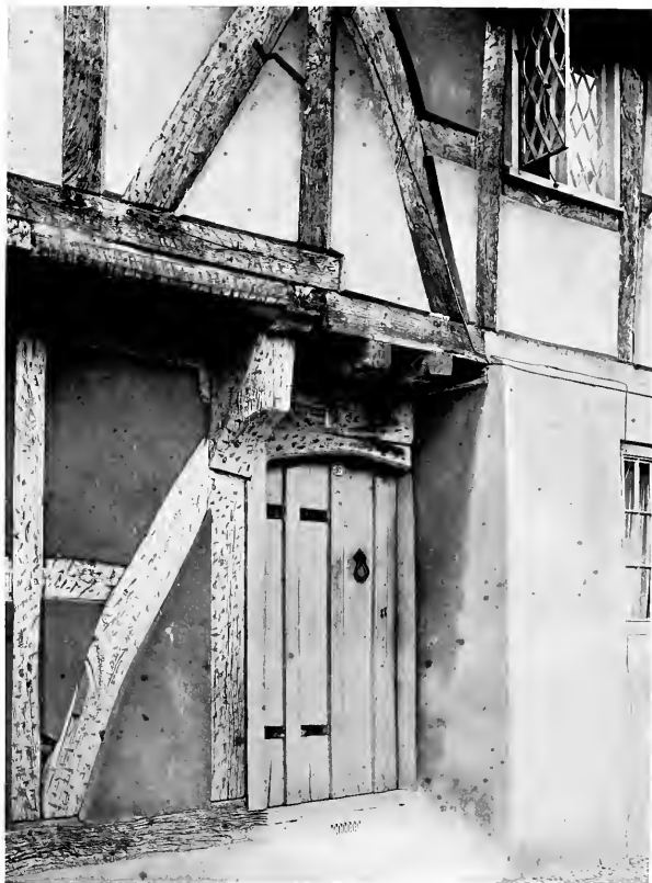
A GROUP OF HOUSES AT HURSLEY, DOORWAY
